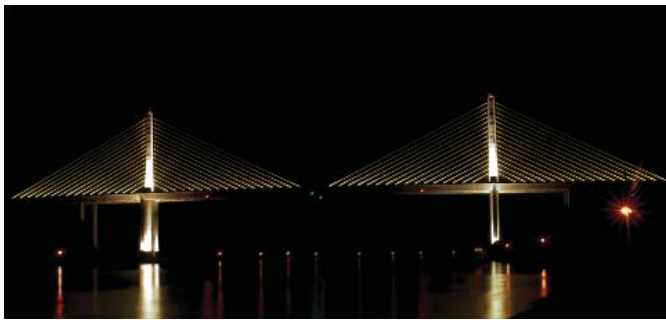
C&D Bridge, Dover Delaware
