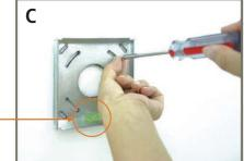
Level the bracket to intended height, install the bracket on the wall.
